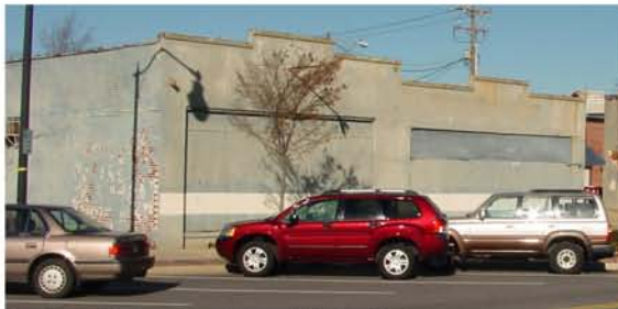
Before Restoration - Main St. View Looking Towards Down Town Greenville
