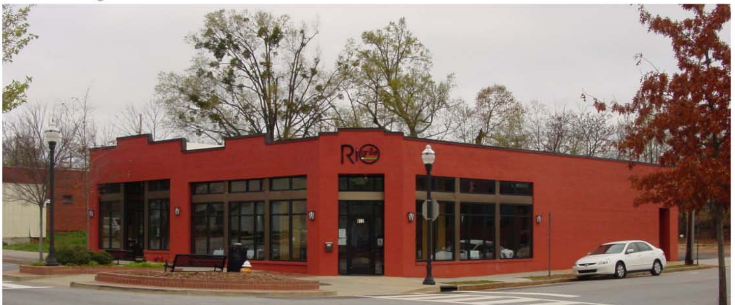
After Restoration and Tenant Upfit - Corner View at Main St. and O'Neal St. Looking Towards the Historic West End of Greenville
