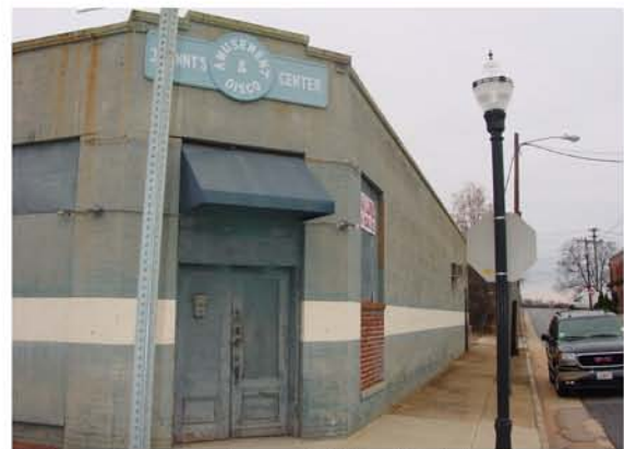
Before Restoration - O'Neal St. View
